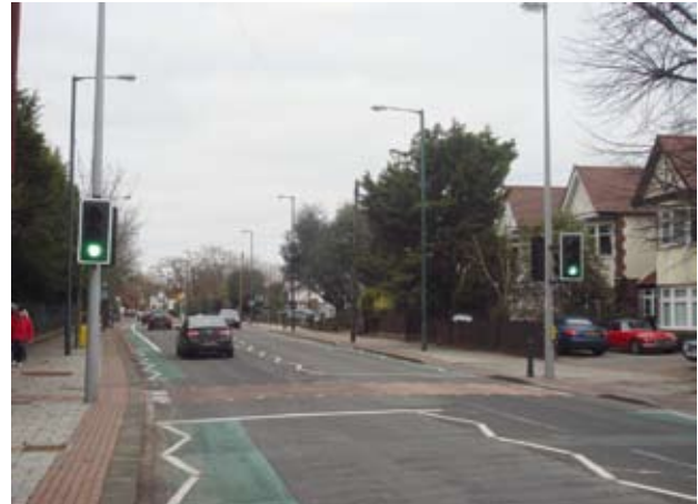
Fig. 3.4 A Pelican crossing where the signal heads have been mounted onto street lighting columns.
