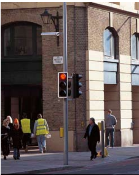
Fig. 3.1 Pelican crossing – signal heads mounted onto existing lamp column to reduce clutter, though a second push button mounting pole is provided, adding to street clutter.
